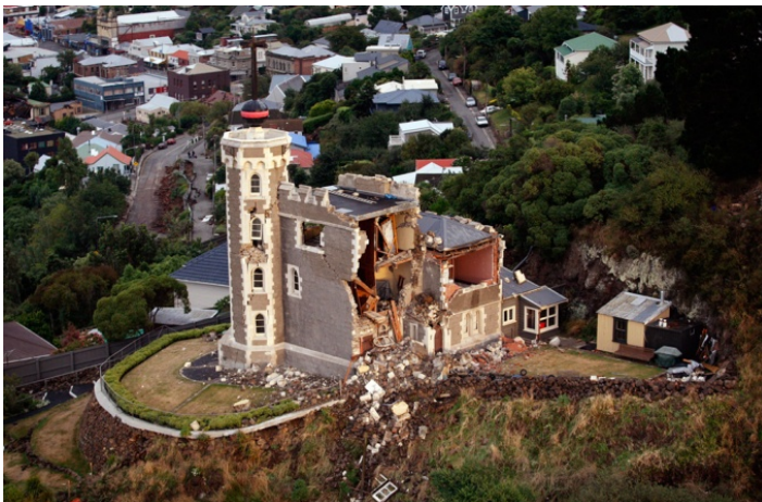
Fig. 30. Topographic Amplification May Play a Role in Damaging an Unreinforced Masonry Building, 2011. http://otilya.com/view/NewsAsia-Pacific/New-Zealand
