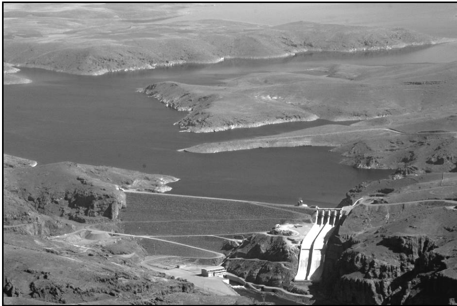
Fig. 11. View of the Ayhanlar dam
