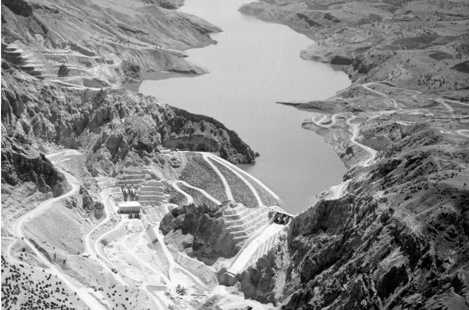
Fig. 7. View of the Kilickaya dam
