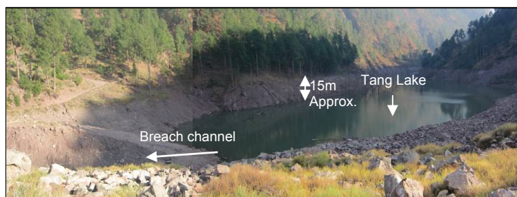
Fig. 12. Tang Lake after breaching (Photo taken on 6 th Dec-2010). From Konagai et al., 2011
