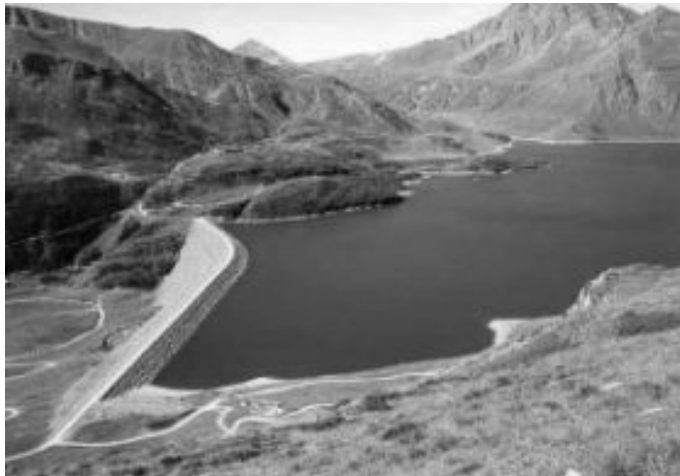
Fig. 13. View of the Boztepe dam
