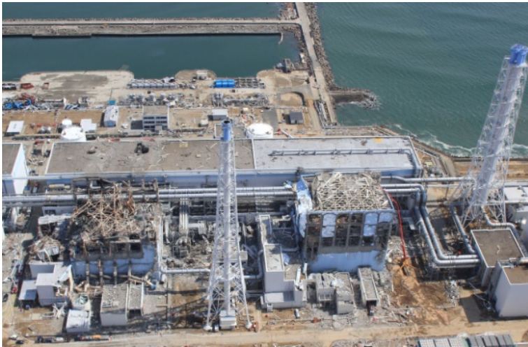
Fig. 34. Blast-Damaged Fukushima Dai-Ichi Nuclear Power Plant Unit 3 (left) and Unit 4 (right). http://pinktentacle.com/
