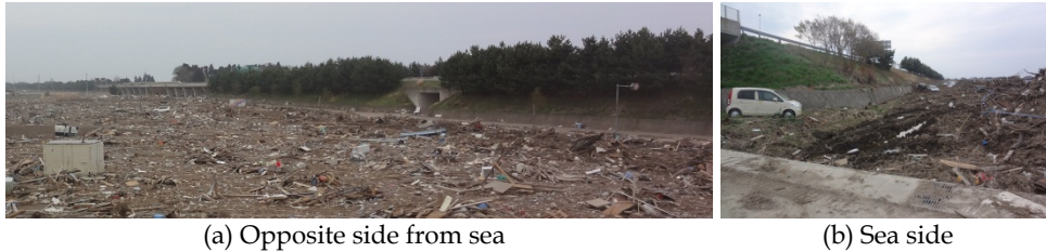
Photo 9. Comparison of damages at both sides of highway embankment
