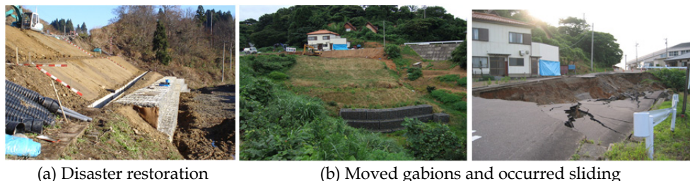
Photo 11. Application of large-scaled gabion at present
