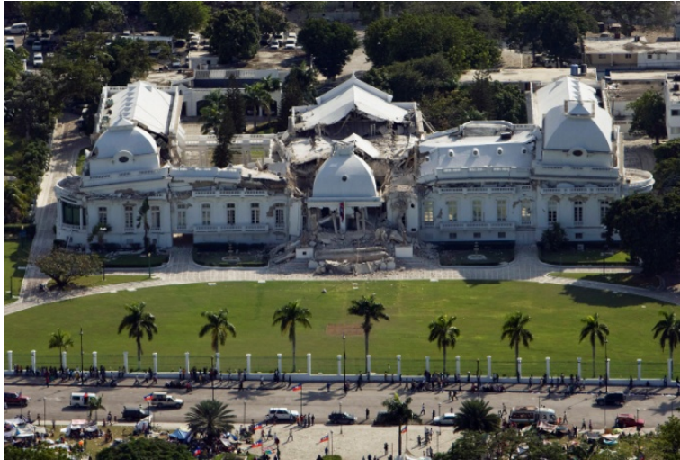
Fig. 20. Damaged Presidential Palace in Port-au-Prince. http://alanrdennis.wordpress.com
