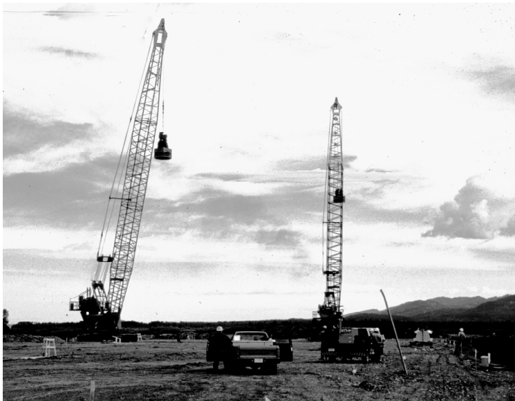
Fig. 6. Deep Dynamic Compaction to prepare a gravelly sand foundation soil for the reconstructed Jackson Lake Dam, Wyoming. Reprinted with permission from Handy and Spangler (2007), The McGraw-Hill Companies, New York.
