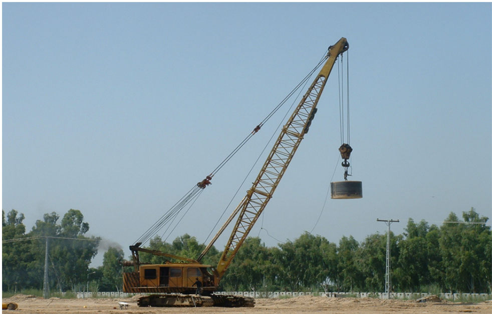
Fig. 3. Dynamic Compaction Equipment (heavy crane, tamper, release mechanism) and process
