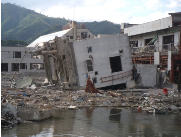
Fig. 38. Overturned Police Station, Onagawa, Japan, 2011.
