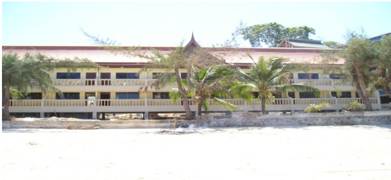
Fig. 41. Building with Crawl Space on the First Floor, Kamala Beach, Phuket Province, Thailand, 2004.
