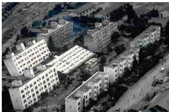
Fig. 1. Apartment buildings at Kawagishi-Cho, Niigata, Japan, tipped after the foundation soil liquefied during the 1964 earthquake.
