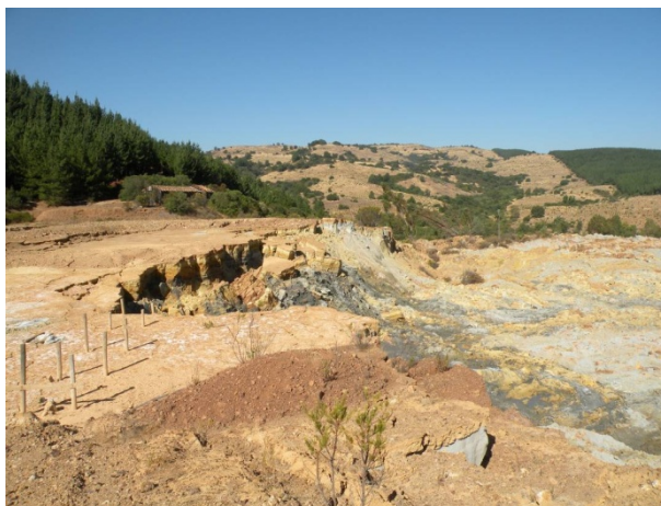
Fig. 24. Upper Scarp of Failed Tailings Impoundment. (GEER 2010)
