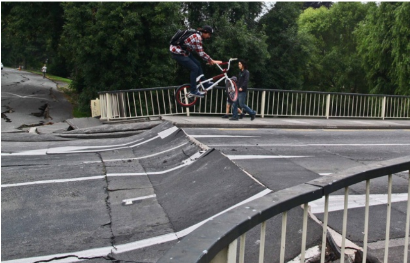
Fig. 47. Settlement of Approach Fill at Bridge Abutment Formed a Bike-Jump for a Youngster. http://otilya.com/view/News/Asia-Pacific/New-Zealand
