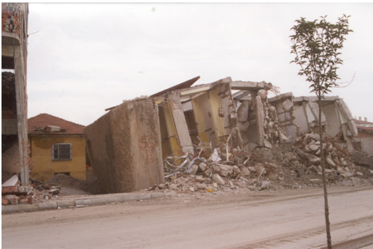
Fig. 45. Overturned Building of High Aspect Ratio in Adapazari City, Turkey, 1999.
