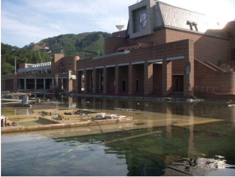
Fig. 33. Waterfront Buildings in Onagawa, Japan Inundated by Tidal Water Due to Earthquake Subsidence. http://tectonics.caltech.edu/slip_history/2011_taiheiyooki/index.html
