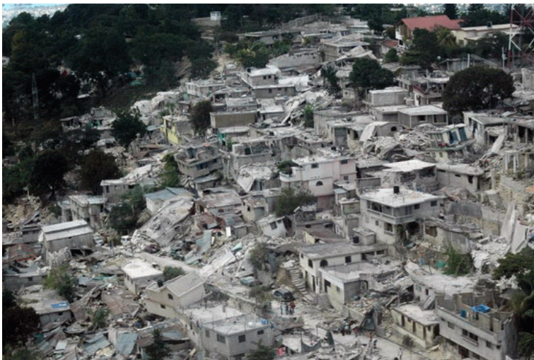
Fig. 19. Damaged Buildings Located on Hill Slope. http://www.worldcatastrophe.com
