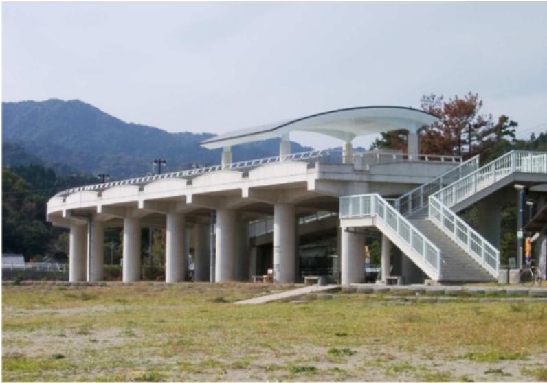
Fig. 48. Vertical Evacuation Structure at Shirahama Beach Resort in Japan. (FEMA 2009)
