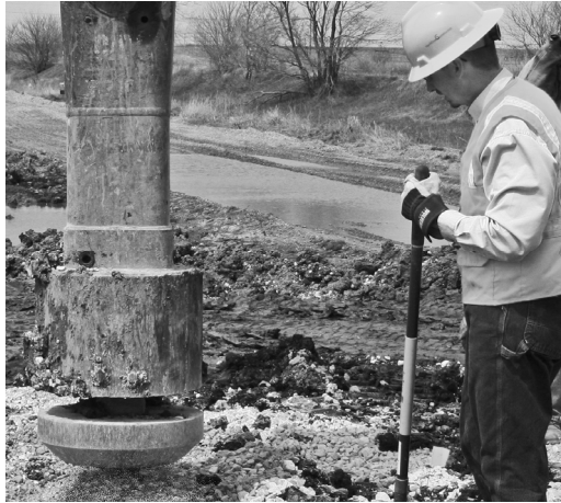
Fig. 7. The Geopier hydraulically actuated rammer is shaped to direct part of the ramming energy outward and increase lateral stress in the surrounding soil.
