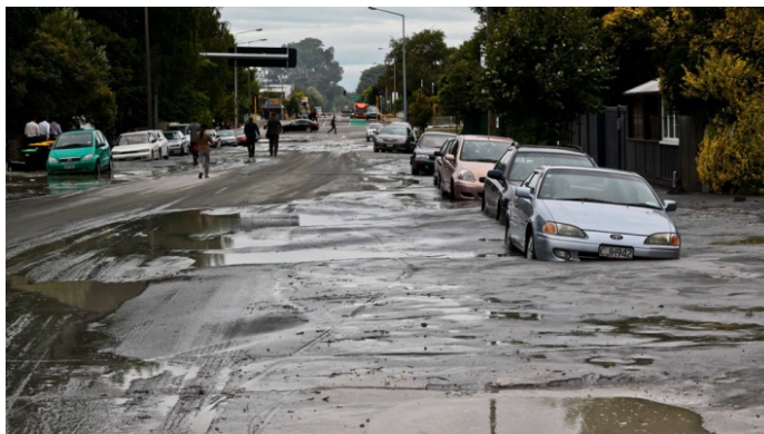
Fig. 26. Liquefied Sand Deposited on Street, 2011. http://otilya.com/view/News/Asia-Pacific/New-Zealand
