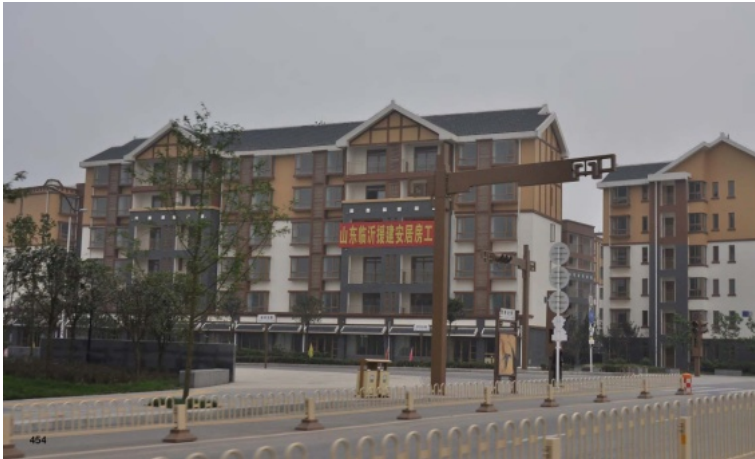
Fig. 18. New Apartment Building Constructed with Support from Linyi City, Shandong Province, 2010. http://www.eeri.org/site/meetings/us-china-symposium
