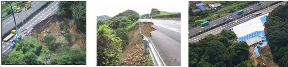
(a) Overview of sliding (b) Shoulder and slope slid (c) Urgent retrieval
