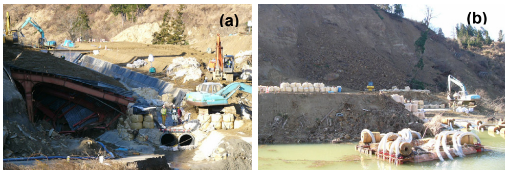
Fig. 4. Emergency works at Higashi Takezawa landslide dam. Photo taken on 20.12.2004 by Takeji & Tadashi, 2005
