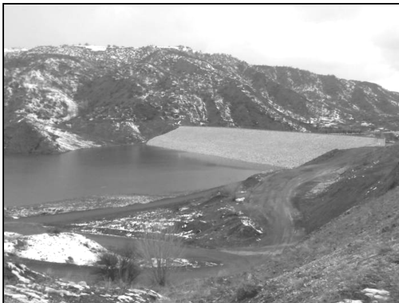
Fig. 9. View of the Hatap dam
